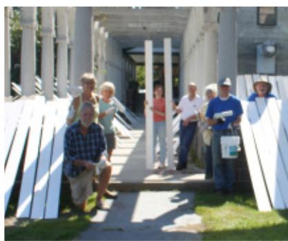
Timber-framing in the East Brethren's Shop has been completed and the reproduction windows have been installed so the building is ready for its new clapboards. The last four Preservation Wednesdays have been spent priming the more than 7,500 board feet of newly sawn clapboards, fortunately the weather cooperated and allowed our volunteers to paint out of doors. It is our hope to have the installation completed before winter.
