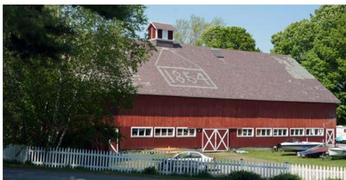
Thanks to two generous grants from **The Lucy and Eleanor S. Upton Charitable Foundation** the slate roof on the 1854 Cow Barn, with its distinctive color and date has been completely restored. In addition, we were able to restore and repaint the ventilator (cupola).
