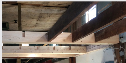
Restored timber framing, note the dark joists on the right. These original joists were found in the attic.
