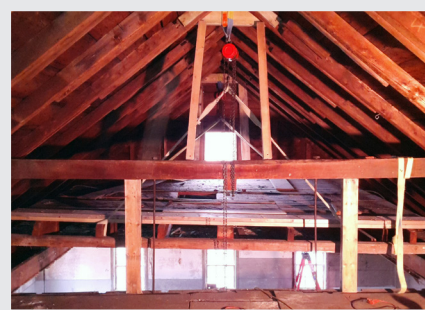
Chain fall in attic of Brethren's West Shop with plaster ceiling being lowered into place.
