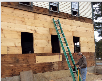
Resheathing of east end of Brethren's West Shop completed in the spring of 2016.
