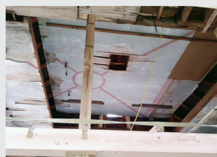
Plaster ceiling being lowered into its original position. Victorian stencil pattern partially visible.
