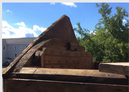
Original cellarway framing on the East Brethren's Shop.
