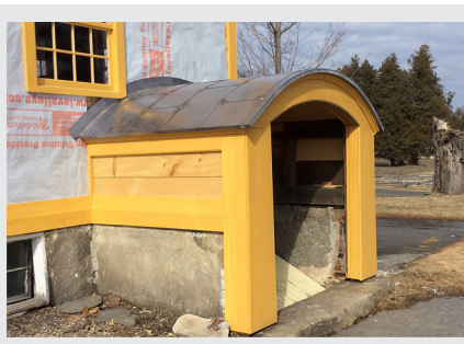
Newly reconstructed cellarway on the East Brethren's Shop.
