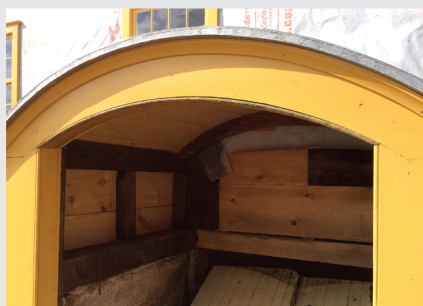
Original arched cellarway door frame on East Brethren's Shop.
