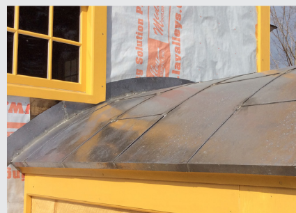
New leaded copper roof on East Brethren's Shop cellarway.
