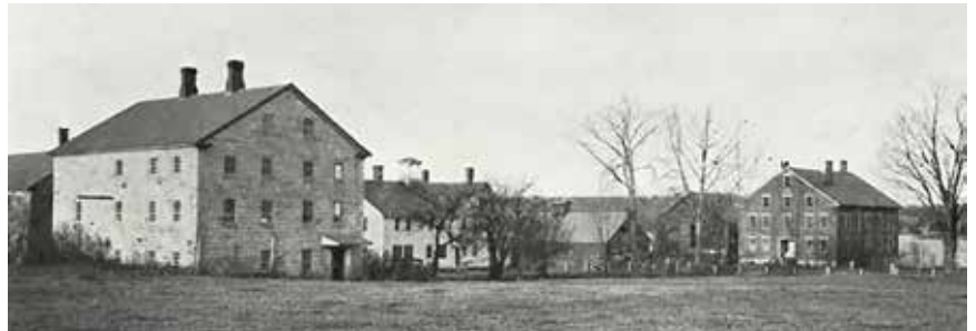
North Family Laundry & Dairy (1831), Dwelling House (1811), Cow Barn (1816), Office Barn (1846), Trustee’s Office (1853).
