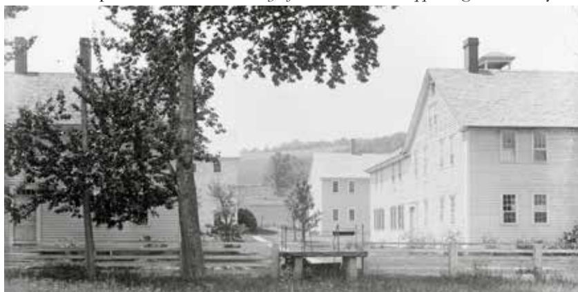
North Family Sisters’ Shop (1818), Laundry & Dairy (1831), Wood House (1844), Dwelling House (1811).
