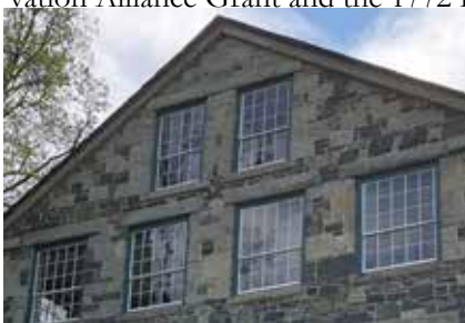
Phase I of Stone Mill Building window restoration.
