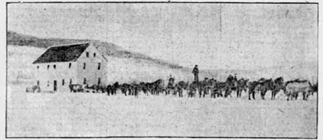
Newspaper account of moving a Shaker building across Mascoma Lake on the ice. April 9, 1905, Boston Daily Globe.
