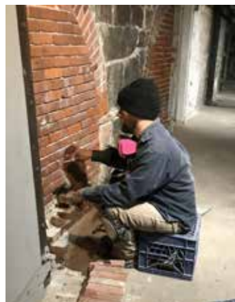
Jeremy Brown at work restoring brick.
