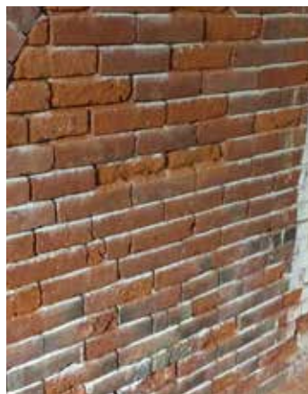
Original soft-fired brick before restoration.
