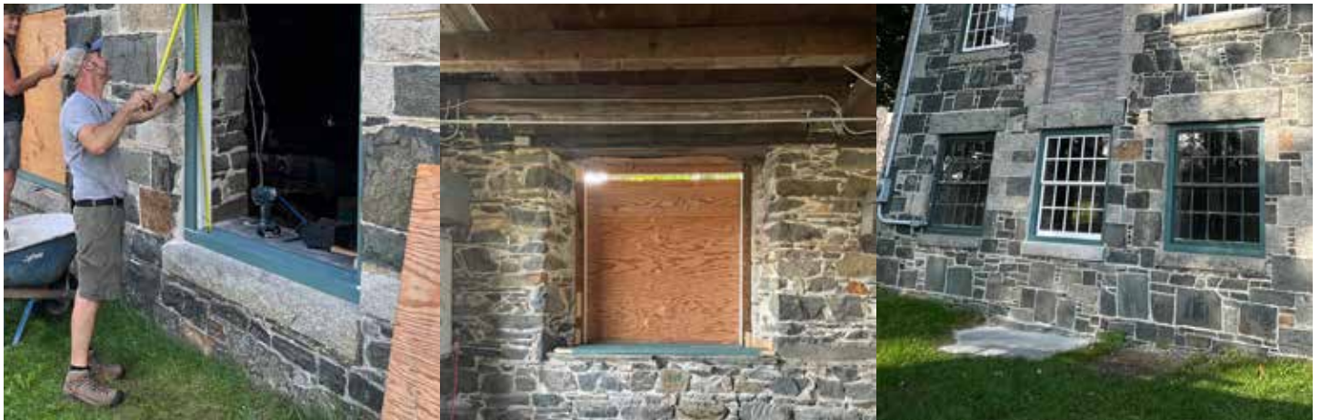
Left to right: David Lewis measures a window opening in the Stone Machine Shop, interior shot of restored basement window opening, and exterior view of restored window opening.
